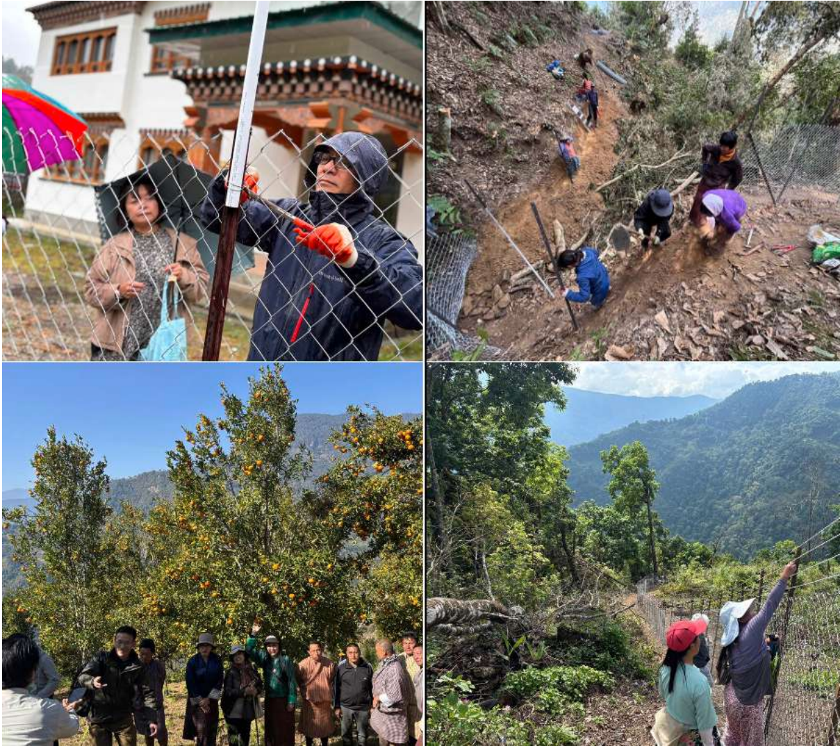
Figure 7.2. Installation of Universal Hybrid Fence at Three Sites
