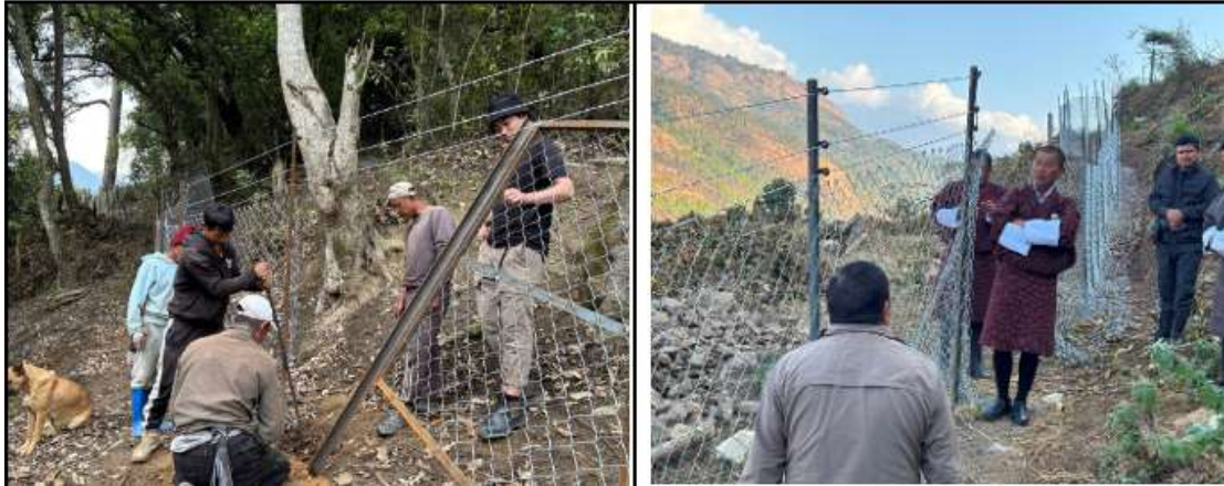
Figure 7.1. Installation of Universal Hybrid Fence
